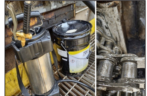
720 CCG being applied to the chains.
